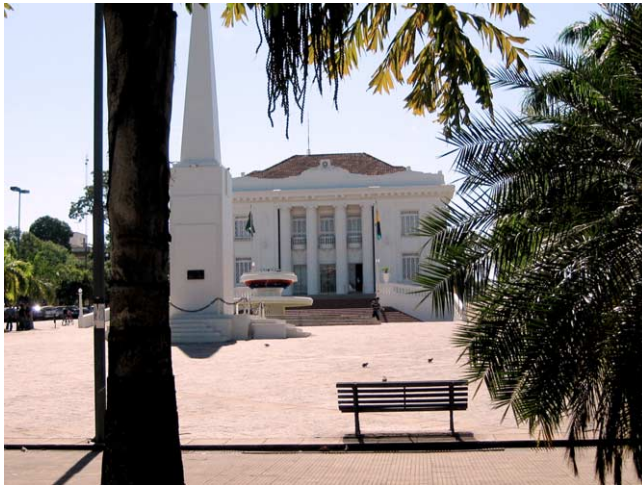
Figure 3. A symbol of Acre's illustrious past: the recently renovated Governor's Palace, originally built in 1930, Rio Branco, Acre. Photograph by Carlos Valério A. Gomes.
