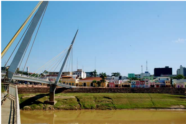
Figure 6. Recently renovated trading and counting houses celebrating Acre's rubber tapping past ("the old market") meets bustling downtown Rio Branco. State of the art pedestrian suspension bridge takes forest citizens back and forth across the Rio Acre bridging the old and new business districts. Photograph by Carlos Valério A. Gomes.
